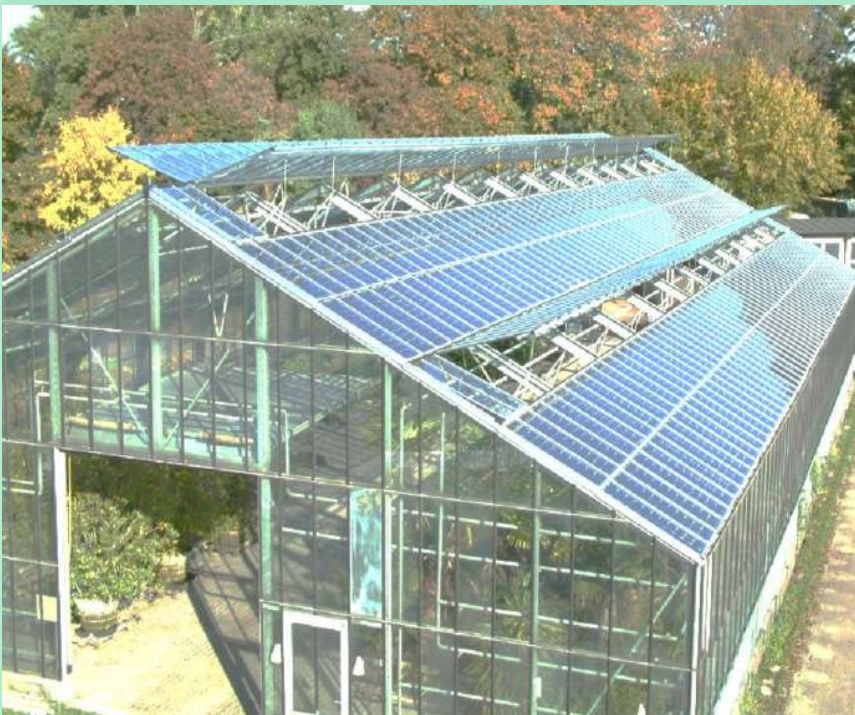
Solar PV Modules and Greenhouse System
